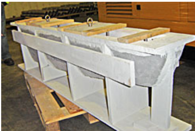
The keel mould is complete
