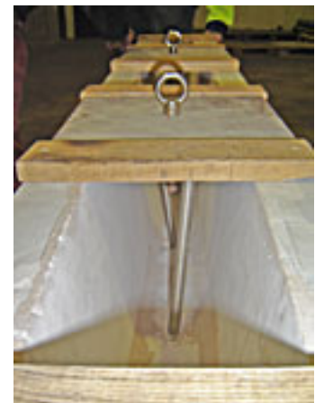
Stainless tubes for the keelbolts
