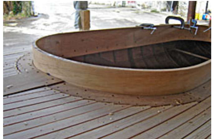
The decks and coaming in place
