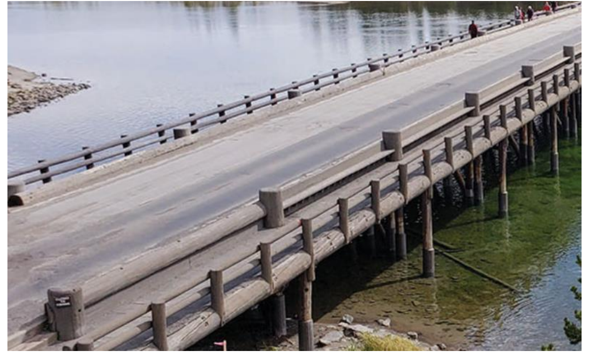
Similar Piling Rehabilitation Works (Ref: Denso Website)
