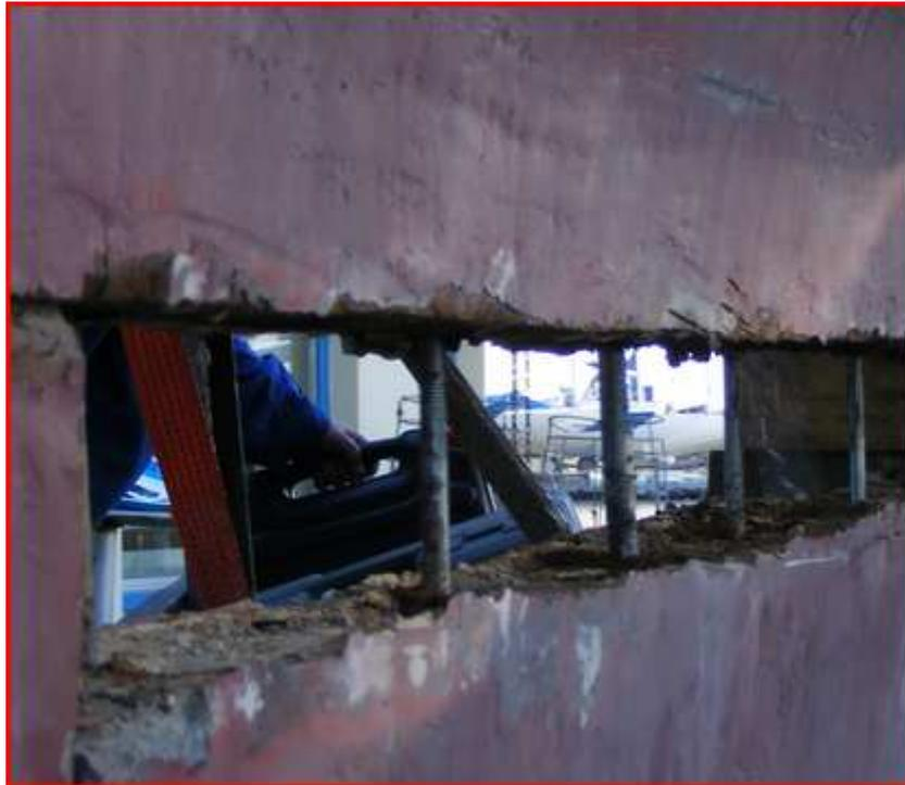
9. In order to retain structural integrity each short bolt was removed and replaced with a new bolt, before the next old short bolt was removed. Because the floors in Rosemary were bronze, the new bolts were made from smooth bronze bar (imperial) purchased in the UK. The bar came with UNC nuts and we threaded it with a UNC die. A twist of caulking cotton was
