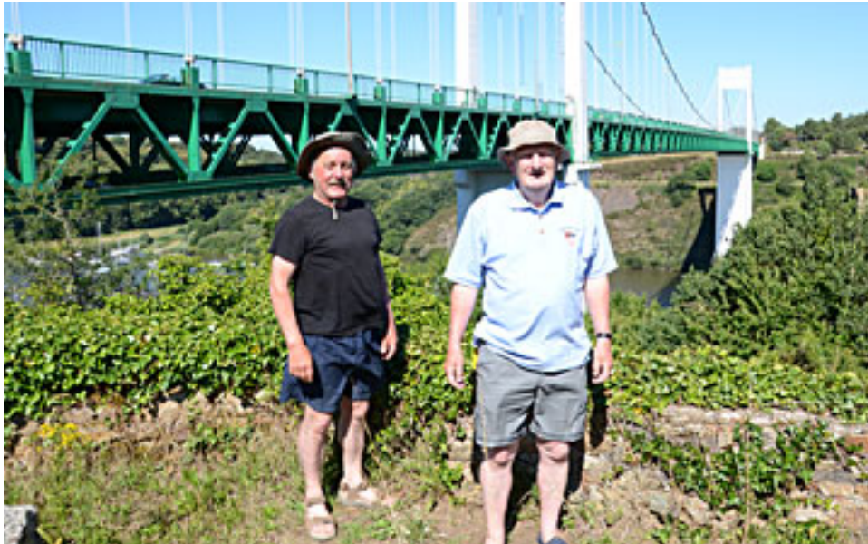
Two motley crewmen checking the suspension bridge (Peter & Seamus)
